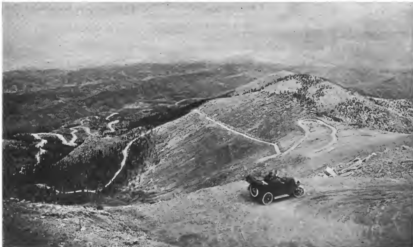
General view showing roadway up Pike's Peak Mountain from a point near the summit. The distance of the hillclimb was 12.5 miles, the maximum grade 10½ per cent, and the average grade 7½ per cent. The sinuous nature of the course is well indicated
